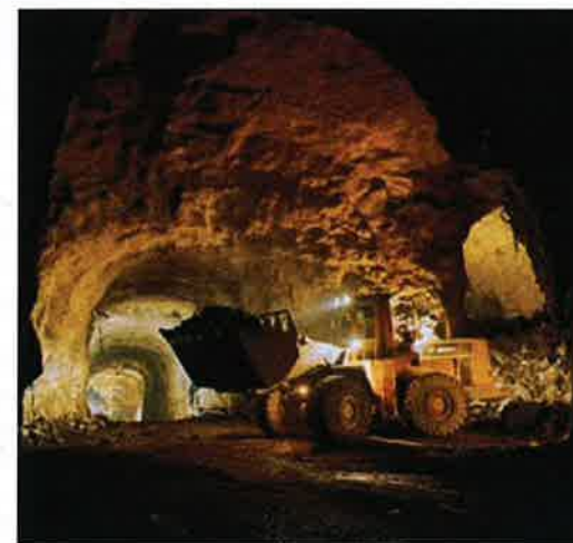
KB's new storage facilities are located 40 meters under the Humlegården park and built in the early 1990's
